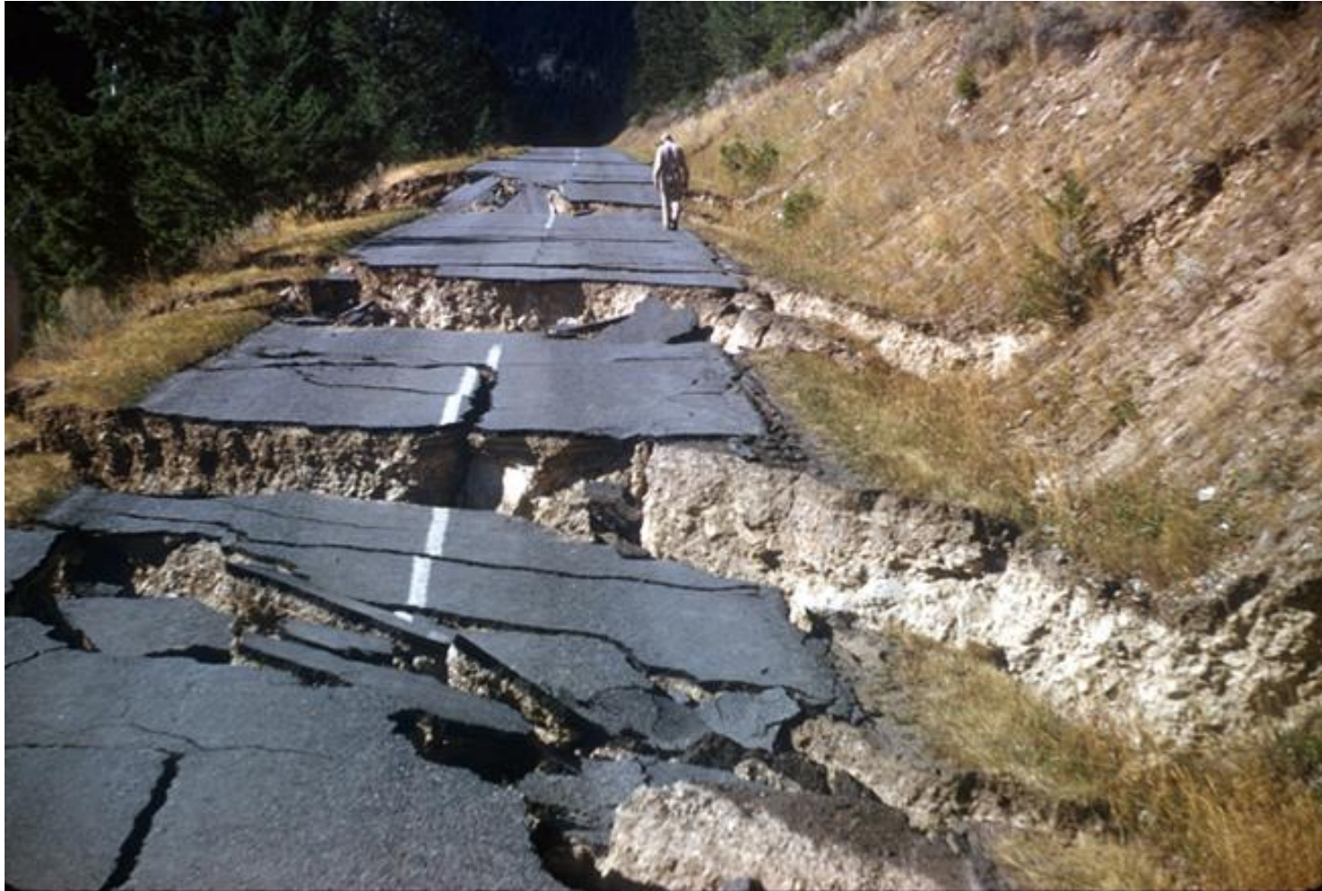
Shaking from the August 18, 1959 magnitude 7.3 Hebgen Lake earthquake caused liquefaction of sediments beneath the road. Photo: R.B. Colton, USGS.
